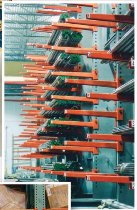
Pipe storage cantilever
