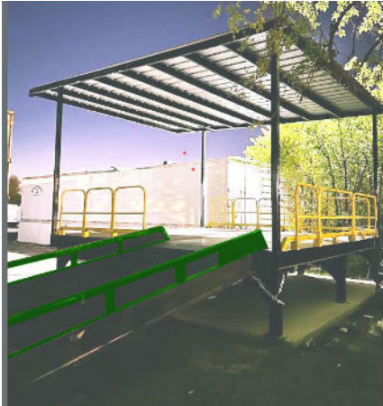
RAMP TO PLATFORM WITH COVER
