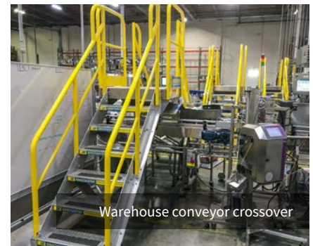
Distribution center machine access
