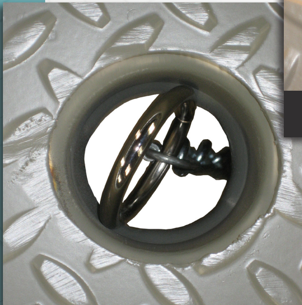
Leveler Chain Cup without Cup Seal
