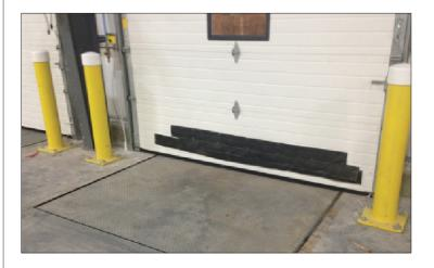
When cleaning in and around the loading dock area, the Mag-Seal can be easily stored on the overhead door. This helps ensure the correct strips stay with the correct loading dock and prevents the Mag-Seal from getting lost.
