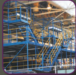
Custom designed access platform
