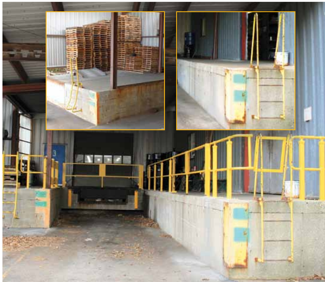
Unprotected ledges (two inset photos) pose a significant safety hazard to workers, which is why Precision Gears turned to Wildeck® to install guard rail on its loading dock (lower photo).
