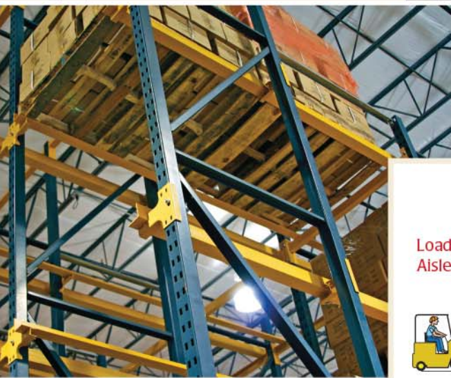
Pallets rest on rails within the bay.
