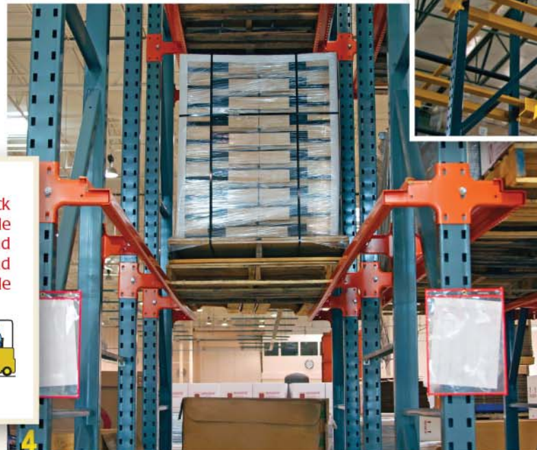
Typical entry view
