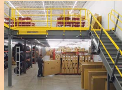
Auto Dealership Mezzanine with Slide Gate
