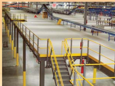
Distribution Center Mezzanine with Resin Board Floor System
