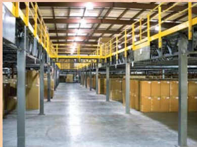
Warehouse Mezzanine with Walkway Bridge
