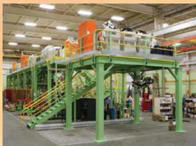
Manufacturing Mezzanine with Gantry Robot
