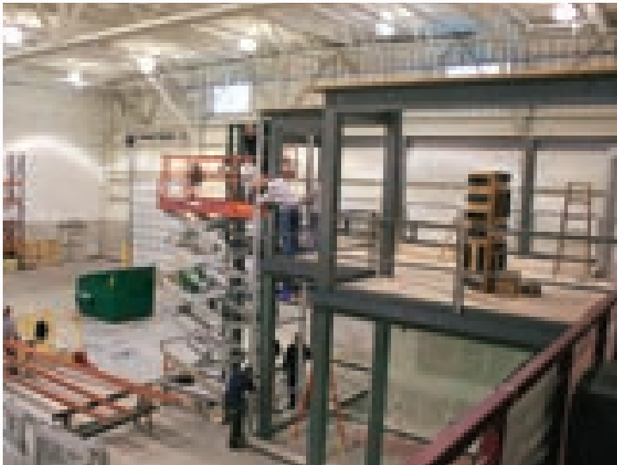
The Wildeck® mezzanine is adapted to meet the needs of the local IUPAT union training facility for glaziers in the hands-on portion of the curriculum. In years past, the training was based in classroom settings only.
