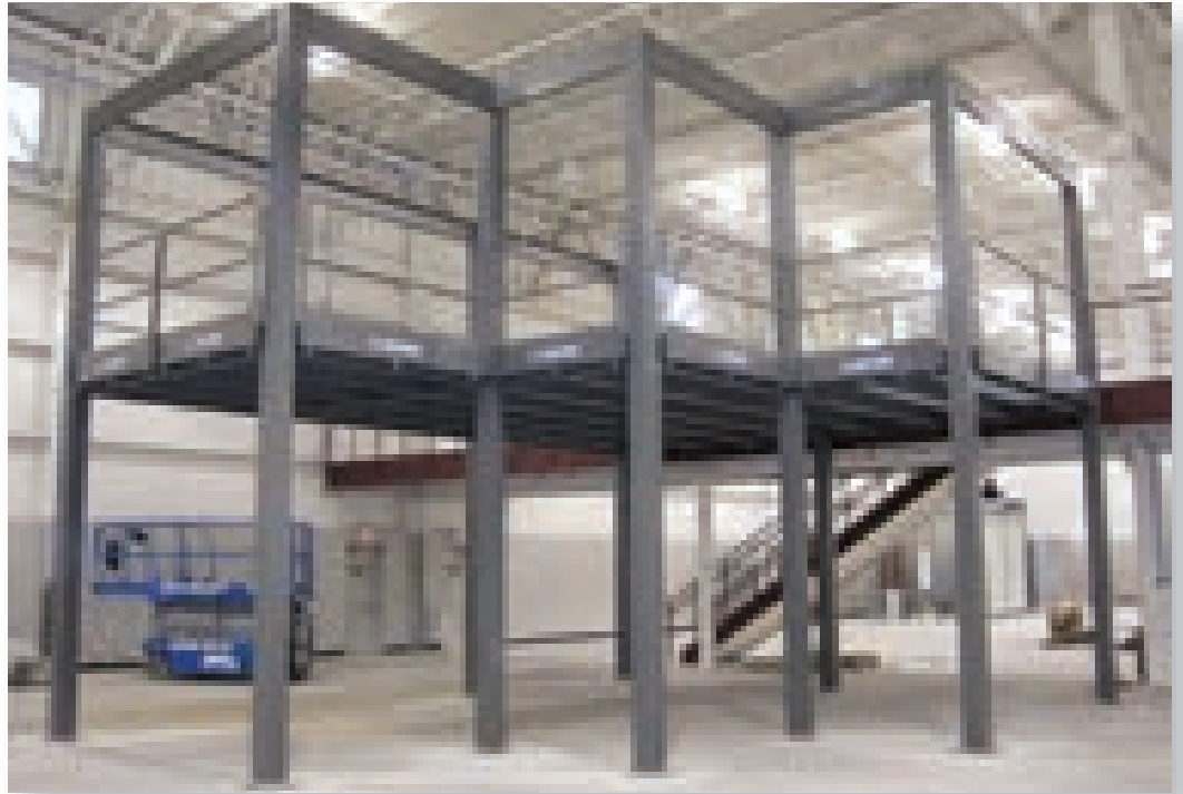
A Wildeck® mezzanine provides an ideal structure for the hands-on portion of the training coursework for IUPAT glaziers. The mezzanine simulates the framework of buildings, and the glaziers use the structure to mount glass door systems and glass curtain walls.
