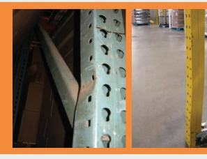
**Note:** Rack welding is not recommended. A proper weld can be difficult to achieve in a warehouse environment and can impact the metal and the rack's load capacity. If damage is not repaired correctly, then this damage can become an issue.
