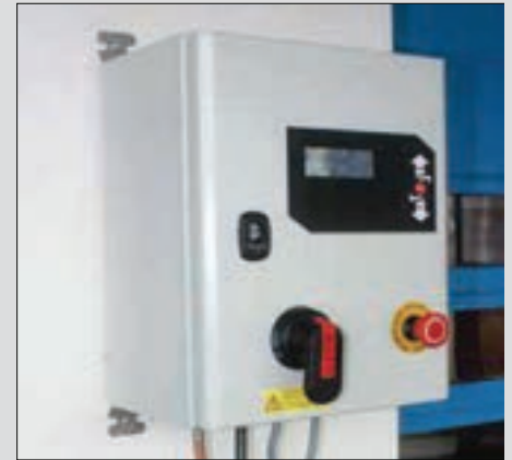
NEMA 4X Smart Start™ NXT control box
